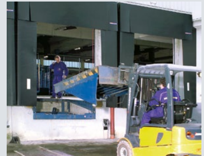
Remove old dock leveller, adjust pit if necessary (e.g. with mounting plates or support brackets)
